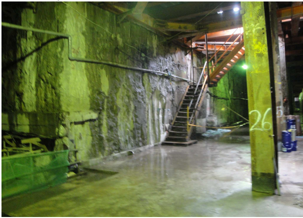
Fig. 3 Quality of diaphragm wall
