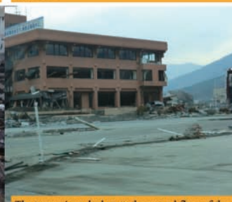
The tsunami reached up to the second floor of the building. Protrudes are seen in the second floor.
