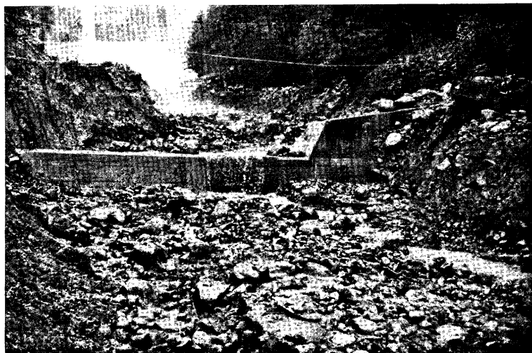
Photo. 2-1. Debris flow running down over dam No. 7 accompanied with dense fog (12 h 50 m , July 13, 1975; Photo. 2-1~2-4 is a series).
