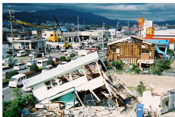
Photo 2 Collapsed houses on the track of tornado.
