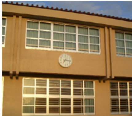
b. Openings installed partitioned sash with thick glass.
