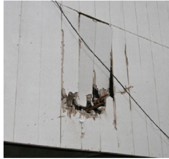
a. Broken walls and openings. b. Break on lightweight concrete wall. c. Falling down of concrete wall.
