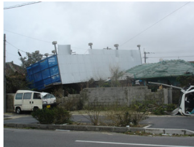
b. Lightweight steel storehouse got upon the neighbouring house.
