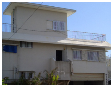
c. Protection with shutters and louvers.
