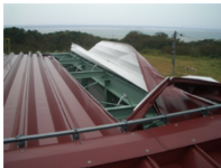
c. Corrugate metal roofing.
