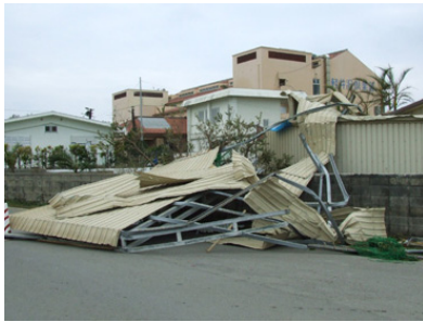
a. Lightweight steel storehouse collapsed.
