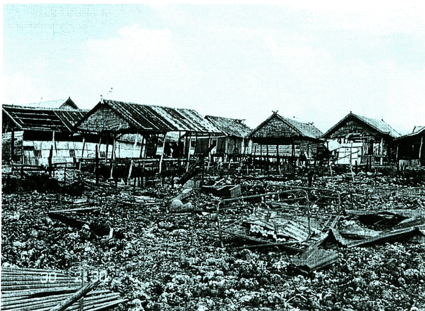
Photo 2 Ruined wooden-made houses of high floor type.
