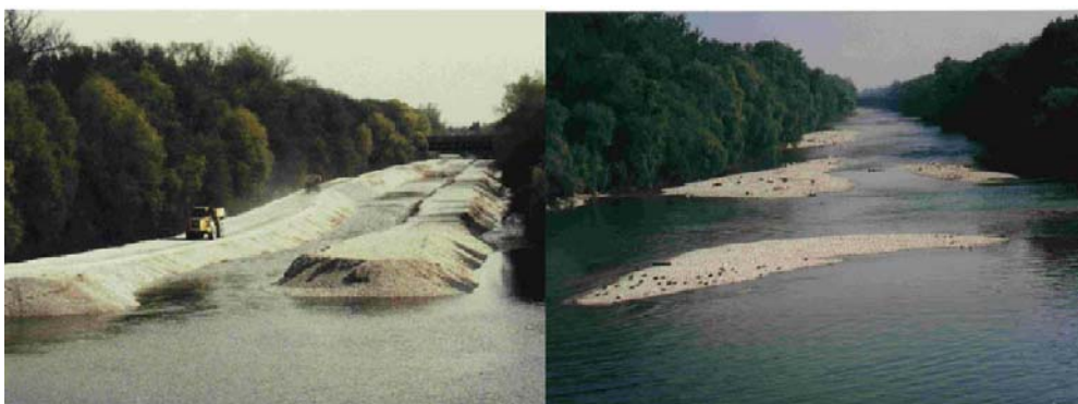
Photo 10 Gravel replenishment into Isar at the Oberfohringer Wehr: Transport of excavated material by truck and deposition in the river bed as depots (left) and naturally distributed gravel material after minor flood events after 3 months (right) (ALPRESERV project)
