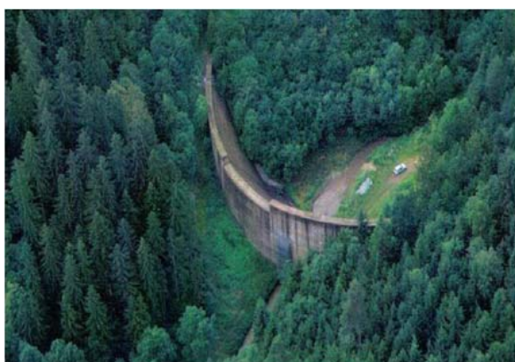
Photo 6 Flood mitigation dam of Ligistbach, Styria, Austria
