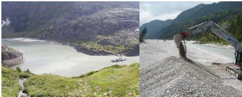
Photo 9 Excavation activities in reservoirs: Suction dredger and floating pipeline at the pilot action Margaritze (left) and conventional hydraulic excavator at Sylvenstein (right) (ALPRESERV project).
