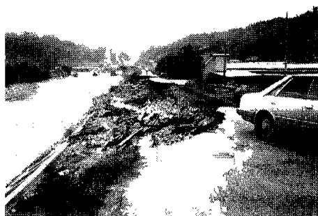
Photo. 2. A eroded levee at the down-stream reach in the Shimoko River.
