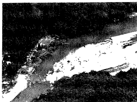
Photo. 3. Whole surface revetment broken completely by overtopping flow.
