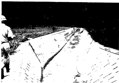
Photo. 6. Slightly damaged revetment in the Aokawa River.
