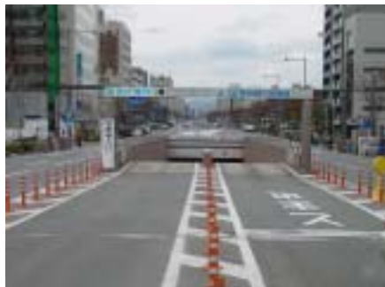
Photo 1 Entrance of underground parking lot
