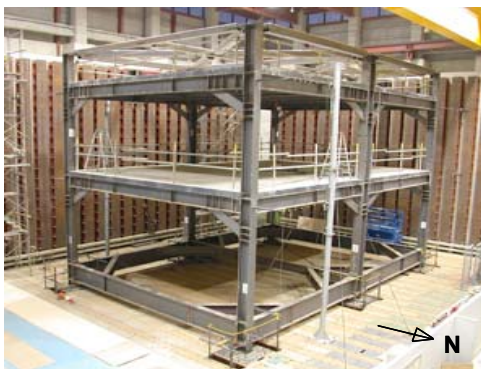
Fig. 11 General view of building specimen
