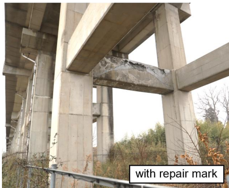
Fig. 1. Damage to middle beams with repair mark, photographed on 18 March 2022.
