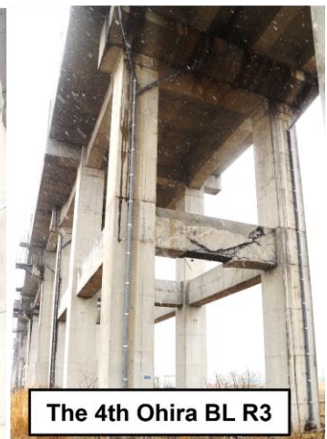
Fig. 2. Damage to two-story RC viaduct at the site of the bullet train derailment, photographed on 18 March 2022.
