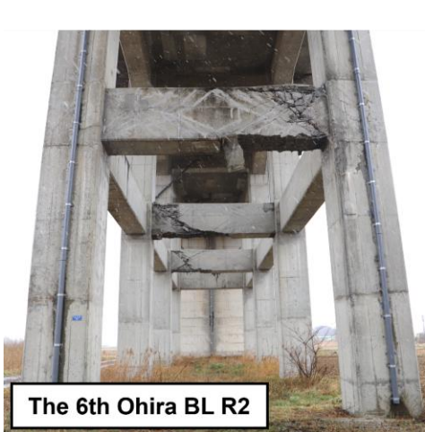
Fig. 2. Damage to two-story RC viaduct at the site of the bullet train derailment, photographed on 18 March 2022.
