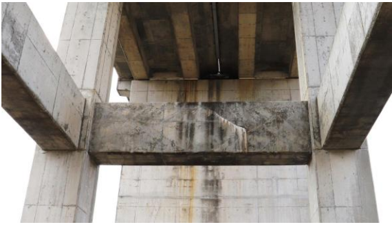
Fig. 16. Actual repair conditions on the middle beams of two-story RC viaduct at the site of bullet train derailment, photographed on 20 February 2021.
