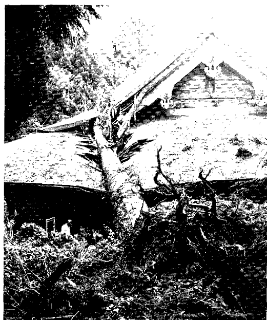
Photo 1 Roof damage by huge tree collapsing from the root (Syakadou at Hieizan Enryakuji-Temple)
