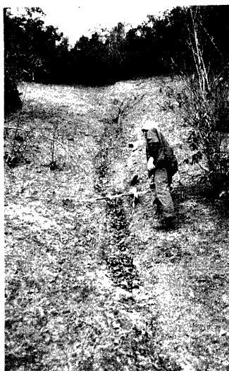
Photo. 1. A surface pattern of a land slide.
