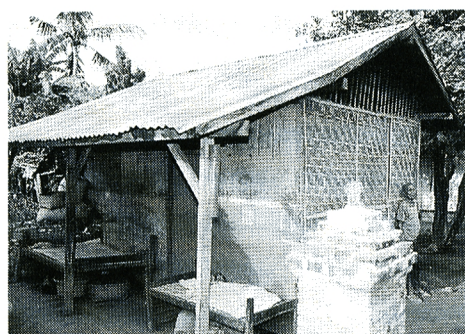
Photo 4 Restoration house at Kalianget village
