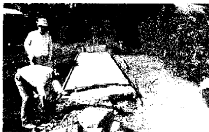
Photo. 2. Damage to a concrete block fence.
