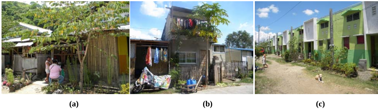
Figure 8.11. Façades of houses in Village 1 (a), Village 2 (b), and Village 3 (c)
