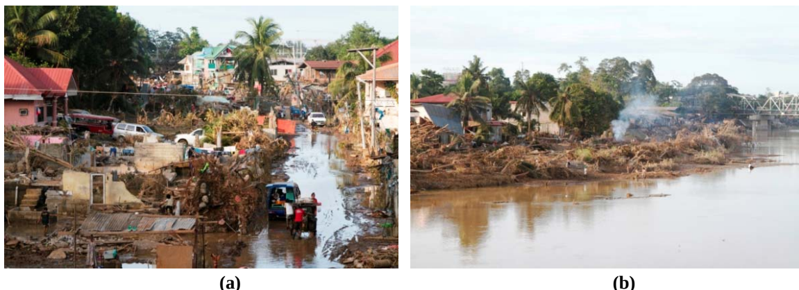
Figure 4.3: (a) Settlements flooded and (b) housing damaged or destroyed by Typhoon Washi
