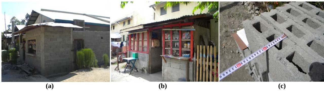
Figure 8.3: CHB wall (a), CHB wall completed with wood (b), and sub-standard CHB (c)
