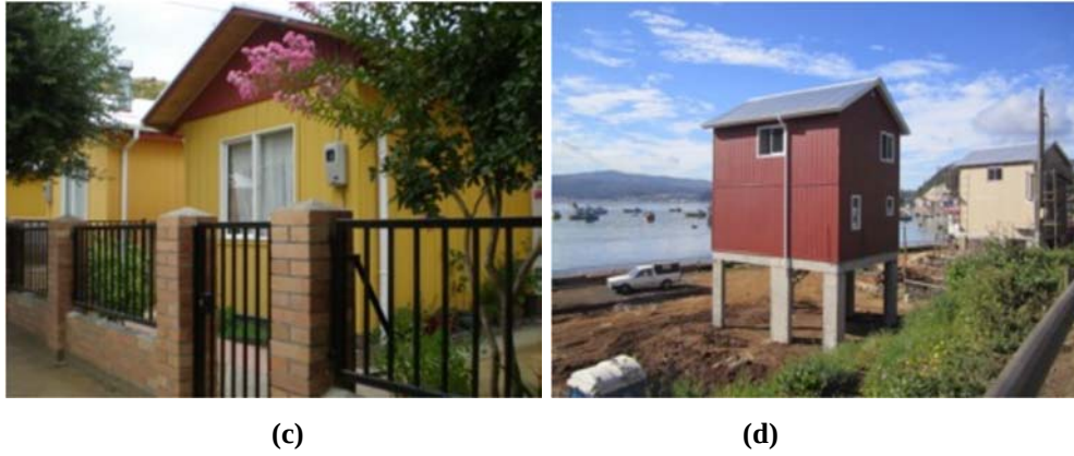
Figure 2.4: Varieties of rebuilt houses (a) Site-built wood house, (b) Site-built masonry house, (c) Prefabricated house. (d) Elevated house.
