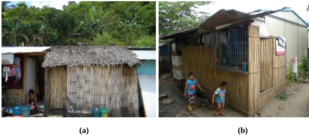
Figure 6.5: Precarious extensions in village 2, using nipa leaves, wood and bamboo (a), and combined bamboo for walls and corrugated galvanized iron sheets for roofing (b).
