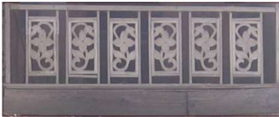
Figure 3.9. Details of Carved Pattern on the Balustrade of a Balcony (1949 Completion)
