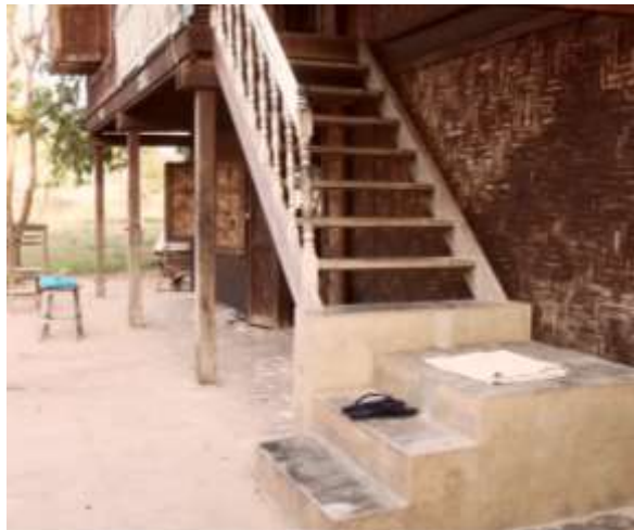
Figure 3.7. Space to Take off Footwear at the Base of a Stair Leading to the Balcony
