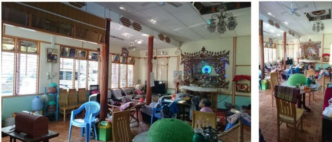
Figure 4.6. Two storey Brick Nogging Building in Chauk (Completion in 2010)
