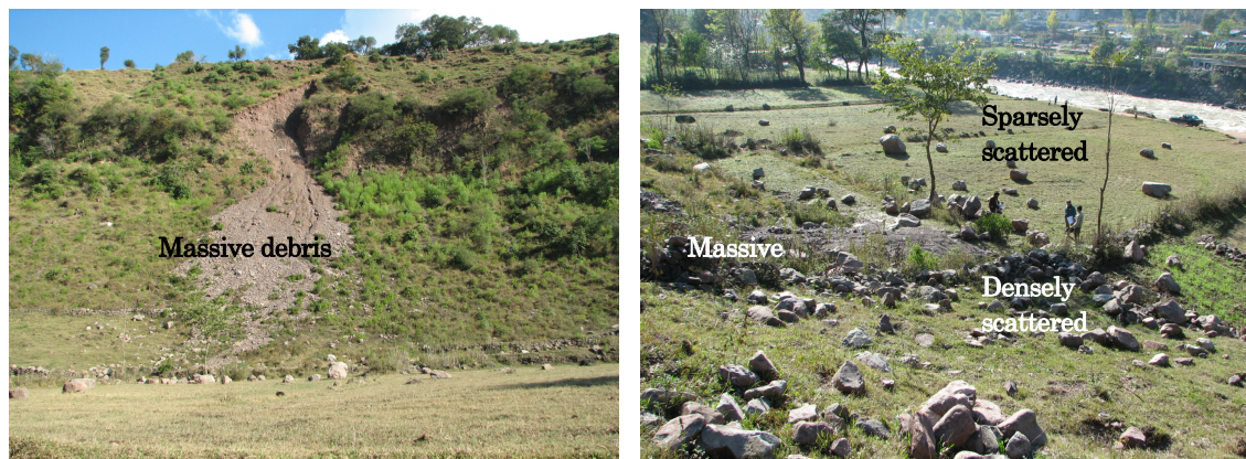
Fig. 5 Slope failures on the terrace scarp of site 7. The depositional area can be divided into three zones by the density of debris: massive area, densely scattered area, and sparsely scattered area. The inclination of the lines connecting these edges and the top of the source area could be used to delineate safety zones
