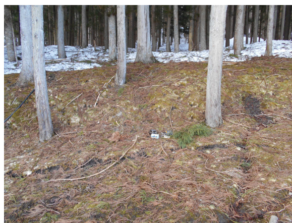
Photo 6 Long step-like crack and a spring point.
