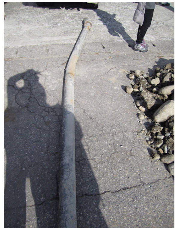
Photo 3 Replacement of water pipe due to the surface fault damage (up-lift about 40 cm).
