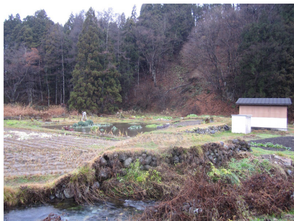
Photo 1 Surface faulting (up-lift about 90cm) at Shiroyama area.
