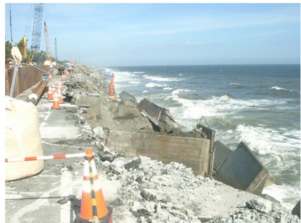
Photo. 3 Storm-induced damage to a stretch of retaining wall of the Seisho Bypass (photograph 16 September 2007)
