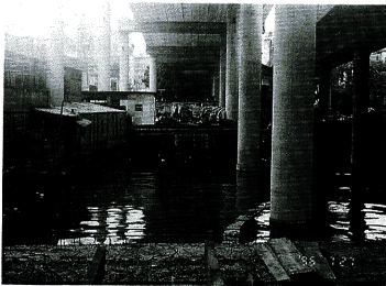
Photo 2 Urban drainage in Guangzhou city
