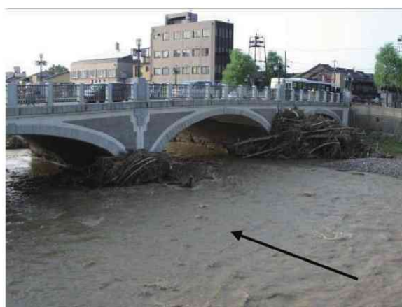
Fig.6 Driftwood captured by Asano Bridge (taken on July 29)
