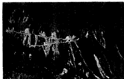
Photo. 5 Many landslips along a road newly built and in a deforested slope.
