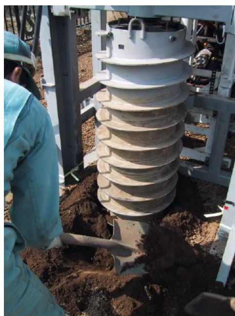
f) Press the drill down with rotation; Removal of the soil on the plane
