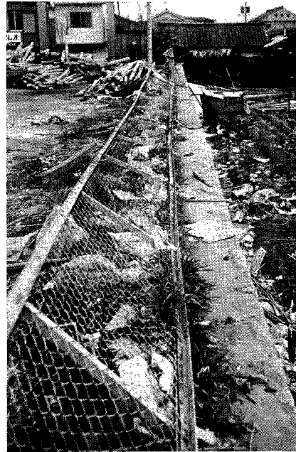
Photo. 6 Damage to a screen fence.
