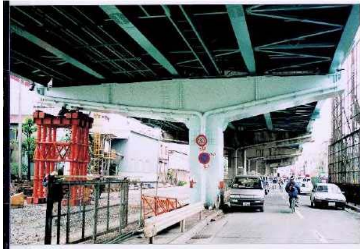
Photo 5.1 T-shaped single column steel bridge pier
