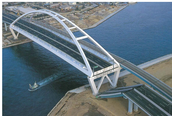
Photo 1.1 A side-span of the Nishinomiya Harbor Bridge fell to the ground
