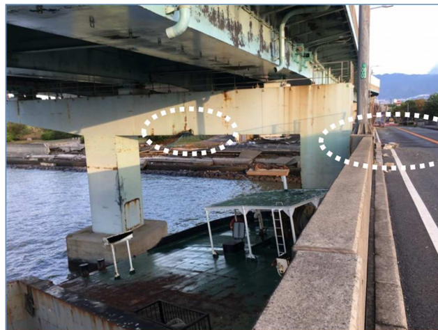
写真 2.2.6.8 橋梁への船舶の衝突 Photo 2.2.6.8 Collision of a ship with bridges
