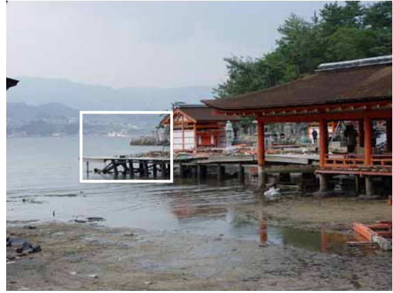
b. Site of collapsed Sagakubou
