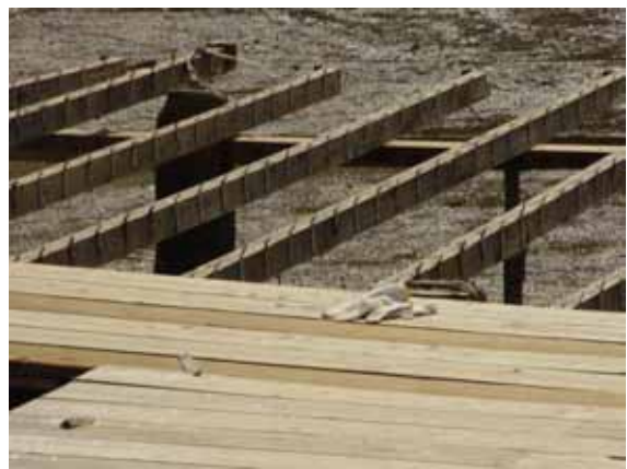
g. Joists and posts of Hirabutai
