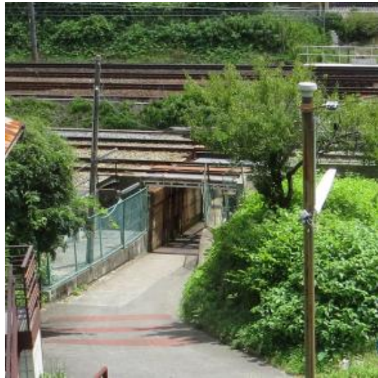
Photo 1 Underpass (passageway under railroad)
