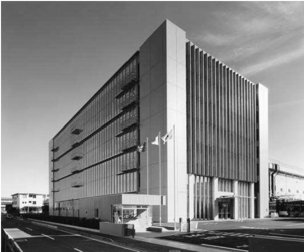
Fig. 1 Photograph of the target building
