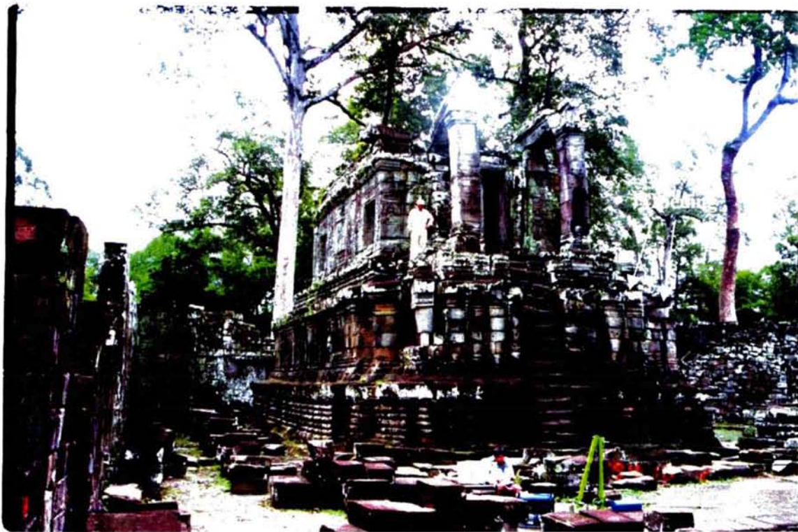
Photo 8-8 North Library, Bayon, front view from west
