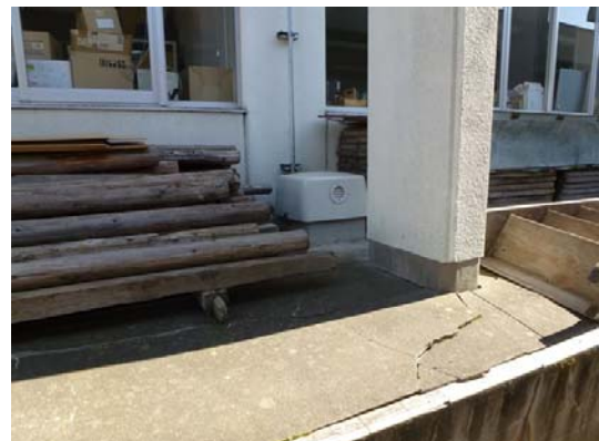
Photo 15 Seismic station at Wakayanagi branch office
