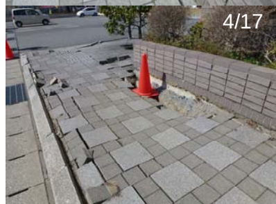
Photo 58 Comparison of the damage of ground pavement
