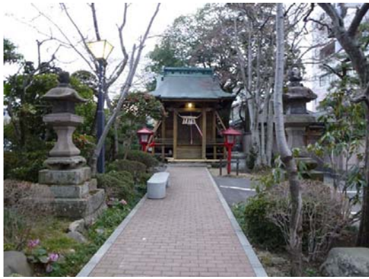
Photo 68 Konpira shrine (after repairing) on 4/18
