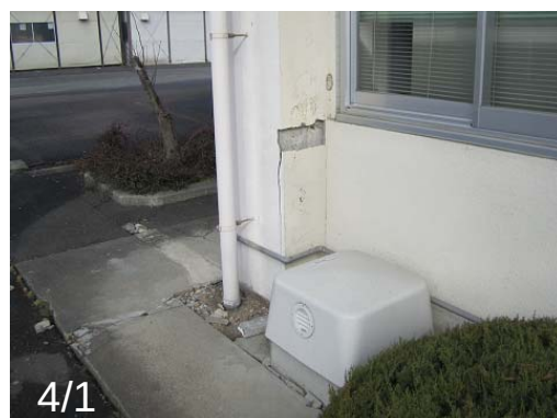
Photo 57 Comparison of the damage of column
