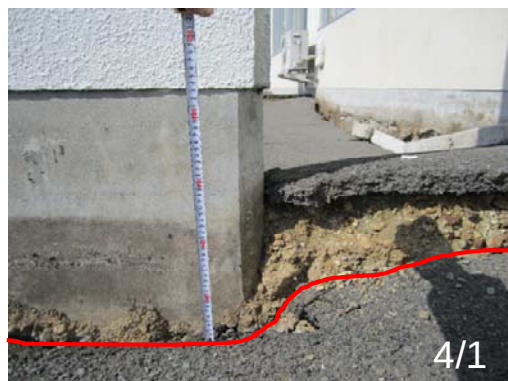
Photo 61 Comparison of the damage of ground pavement
