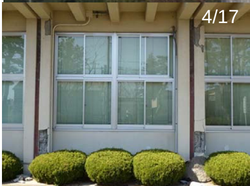
Photo 59 Comparison of the damage of RC column
