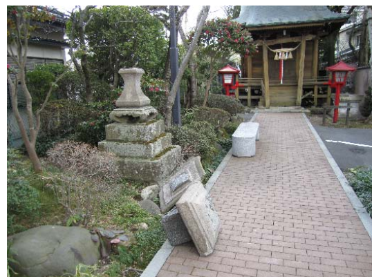
Photo 67 Konpira shrine (before repairing) on 3/31
