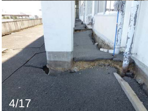
Photo 61 Comparison of the damage of ground pavement
