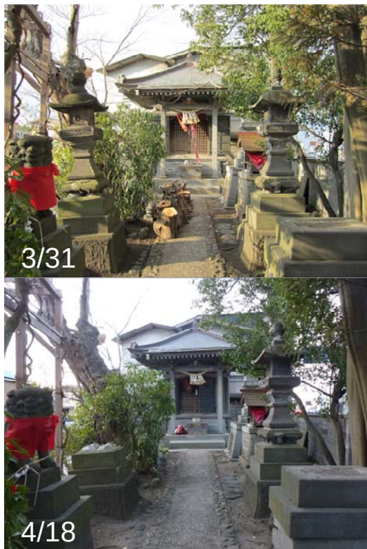
Photo 69 Damage of Kanaya shrine (3/31 and 4/18)
