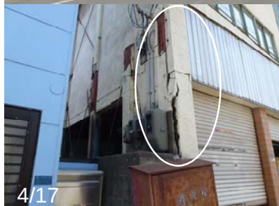
Photo 57 Comparison of the damage of column
