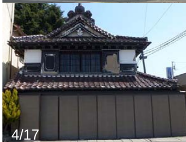
Photo 56 Comparison of the damage of plaster wall
