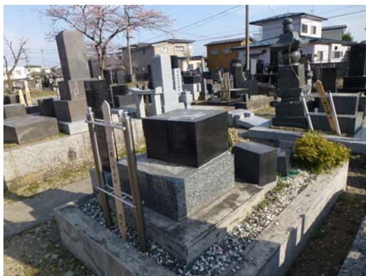
Photo 66 Damage of the graveyard in Zuisen-ji
