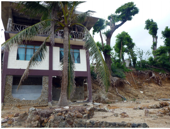
Photo 4 Damaged building and scoured cliff at Pa-on beach resort in Estancia. Clear water mark was observed inside the room of second floor. Stone walls of the first floor are collapsed by wave force.
