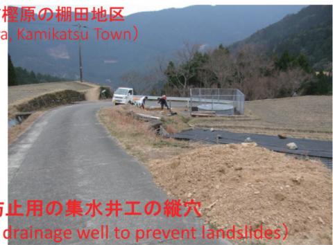
Figure 24: Pit of a drainage well to prevent landslides in Kashihara
