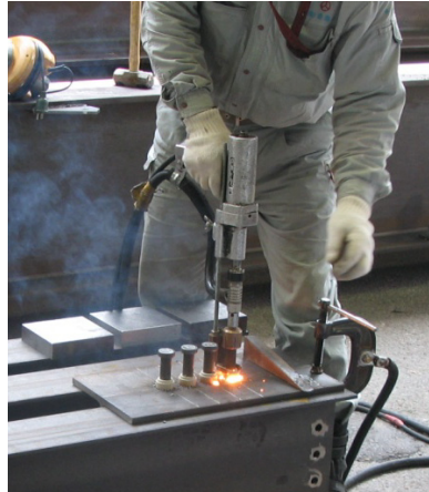
Fig. 5. 2 Welding of headed studs
