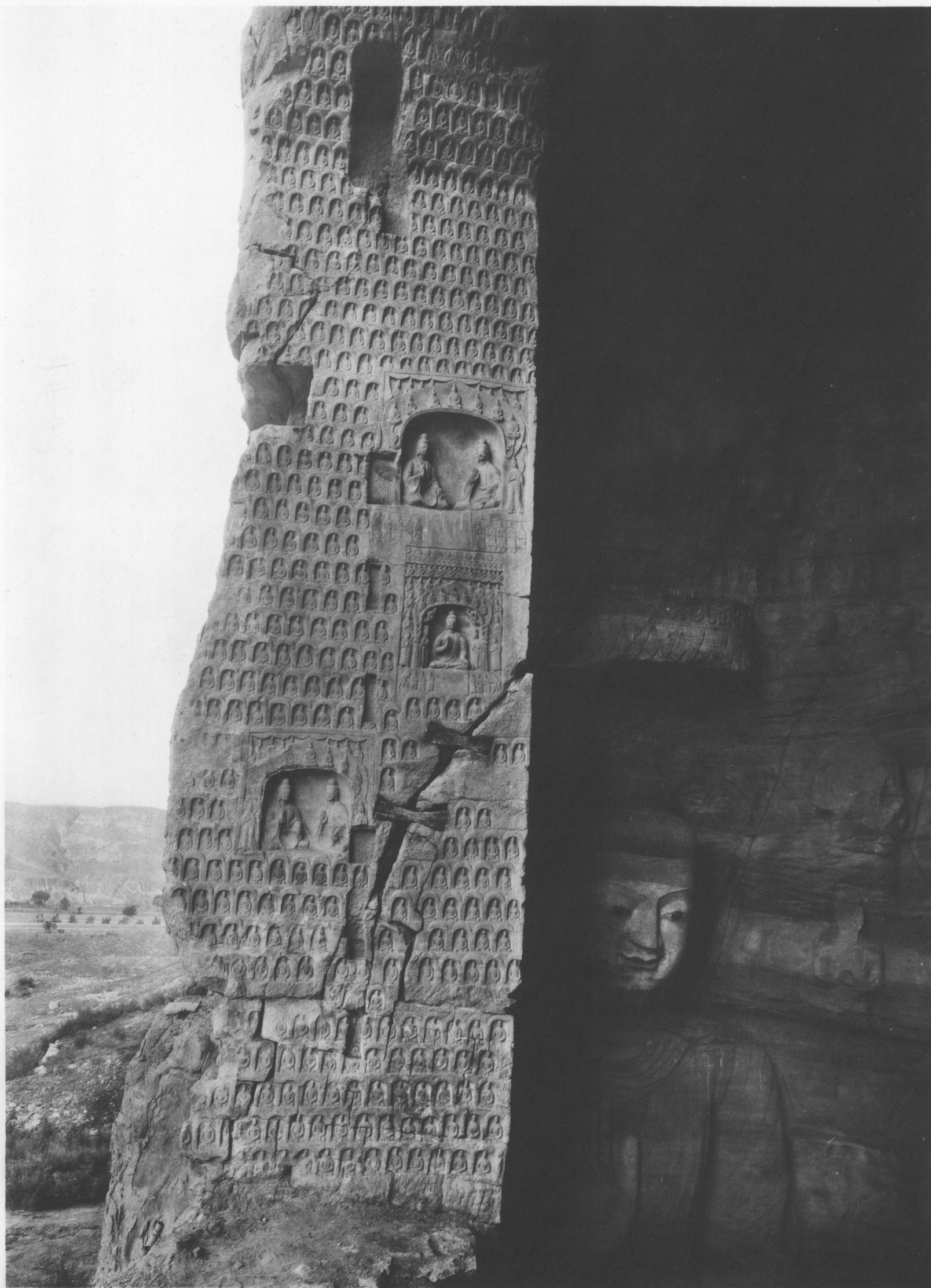
Window, West Reveal.
