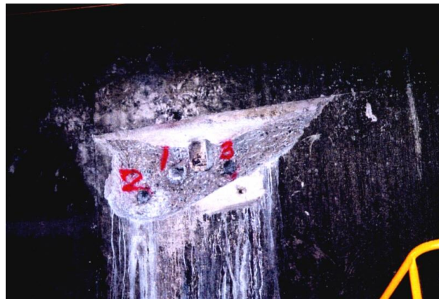
Figure 1 Lining of Fukuoka Tunnel after spalling (Asakura et al., 2001)
