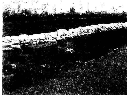
Photo 2 Sand bags stacked on the parapet of the bank of Shonai river
