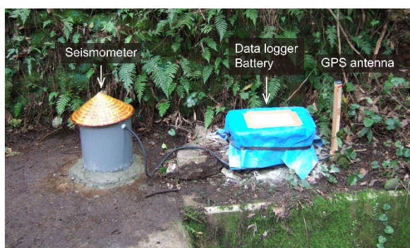
Photo 1 Installation situation of observation equipment at station MK70. The seismometer is installed at the end of a sabo (erosion and sediment control) dam, and covered with a PVC pipe and a sedge hat. The data logger and a battery are stored in a plastic box covered with blue sheet.
