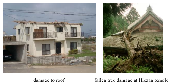
Fig. 10 Investigating strong wind disaster by typhoon
