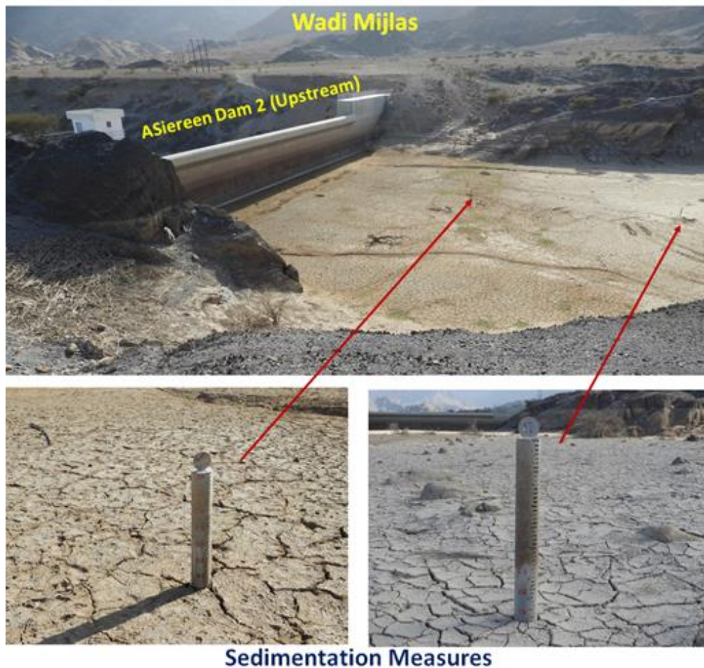
Fig. 9 Sedimentation measures at the reservoir of Asserrin Dam at the upstream of Wadi Mijlas (Photos taken by Kyoto University Team, Field Survey on Nov. 29-Dec. 2, 2017)
