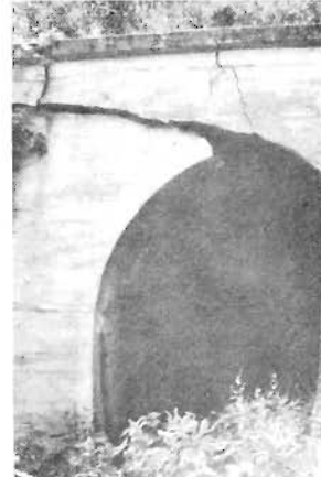
Photo. 4. Eastward mouth of the old Kamenose Tunnel.
