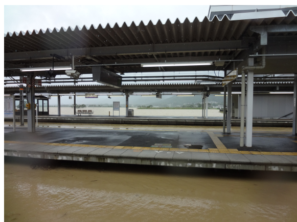
Photo 5 Flood water about reaching the platform of JR Kameoka station
