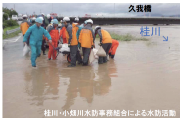
Photo 3 Flood fighting during flood water overtopping area
