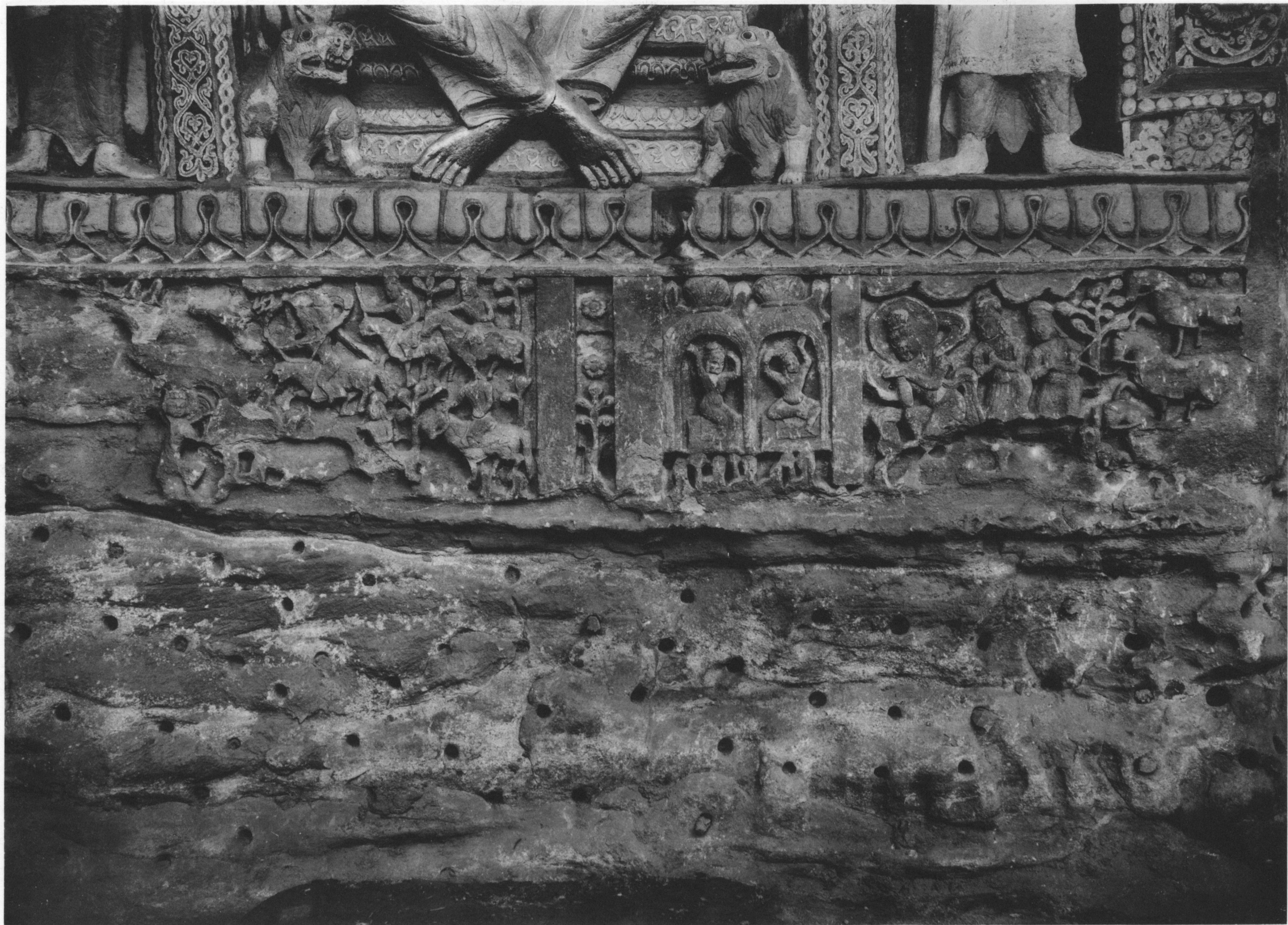
Ante-Room, North Wall, Bottom Storey.
