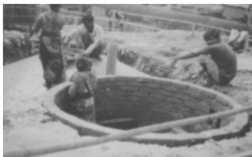
Photo 1 Constructing Bio-gas Plant
