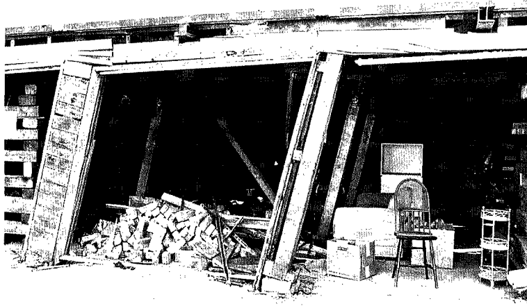
Photo. 8. Failure of soft first storey of an apartment building in Marina District (photographed on 11/10/89).
