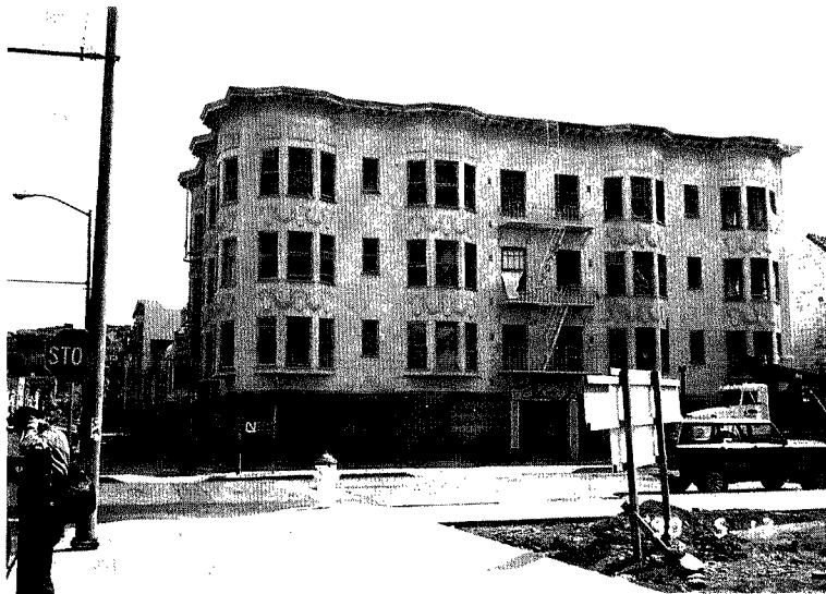
Photo. 9. Apartment building (same as the one in Photo. 7) under repair works (photographed on 5/13/90).
