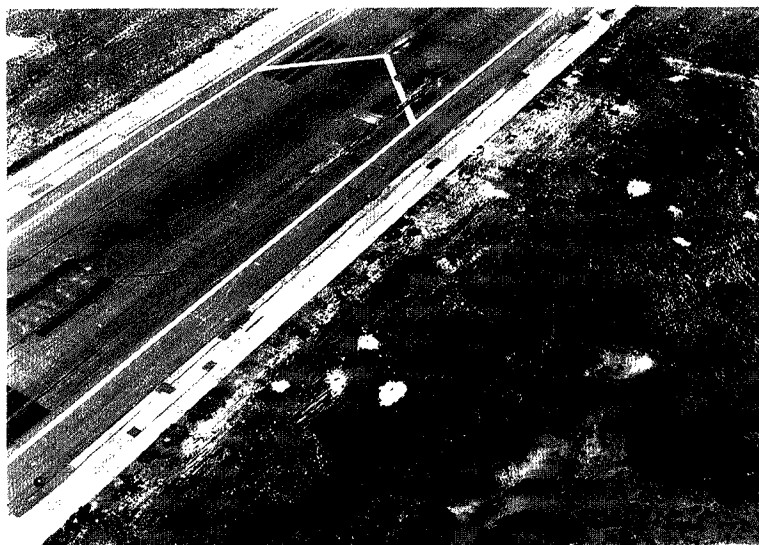
Photo. 5. Sand boils and cracks of runway due to soil liquefaction at Oakland International Airport (photographed on 11/11/89).
