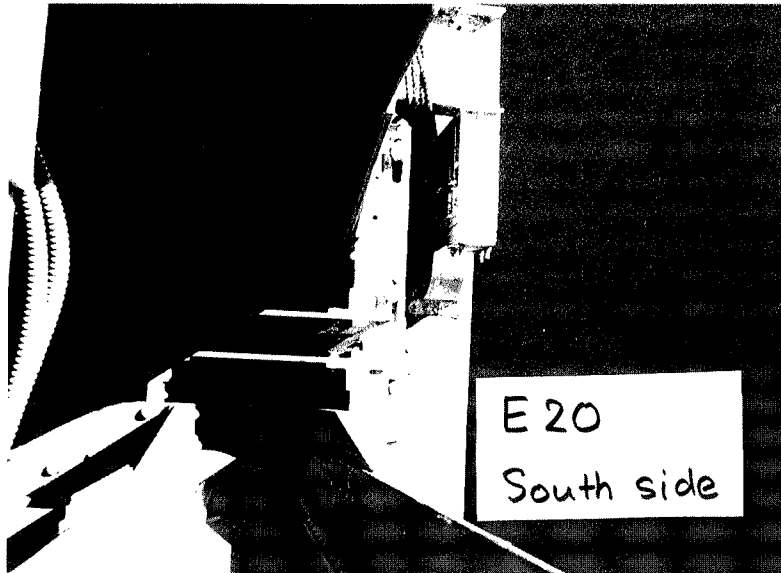
Photo. 20. Deformed restrainer on Pier 20 of Bay Bridge (photograph by A. Astaneh).
