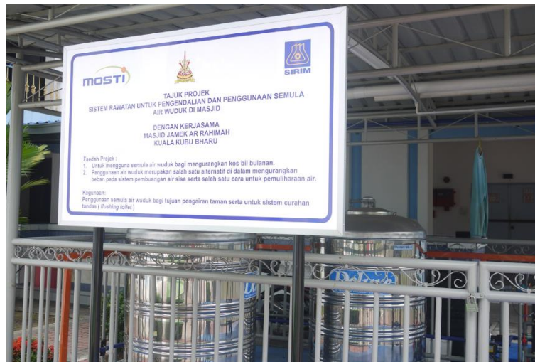
Figure 3.4.2-1 Ablution Water Recycling System in a Mosque in Kuala Kubu Bharu
