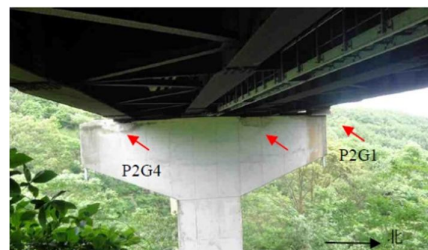
(b) relative displacement between girder and pier
