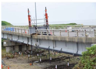
Static load test
