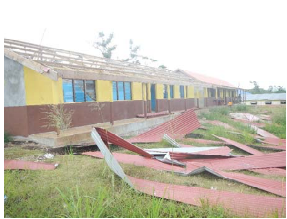
Figure 4. Damages to a school building located in the middle of Tanna island.
