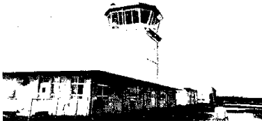
Photo. 4. Damaged control tower of the Ishigaki Airport.
