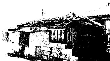
Photo. 9. Damaged tiled roof of a typical Okinawa house.
